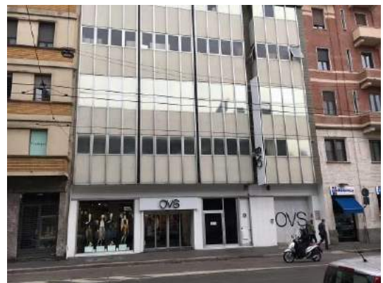
Vista esterna – V. Cuneo
