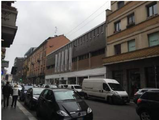
Vista esterna – V. Marghera
