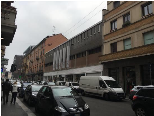
Vista esterna – V. Marghera
